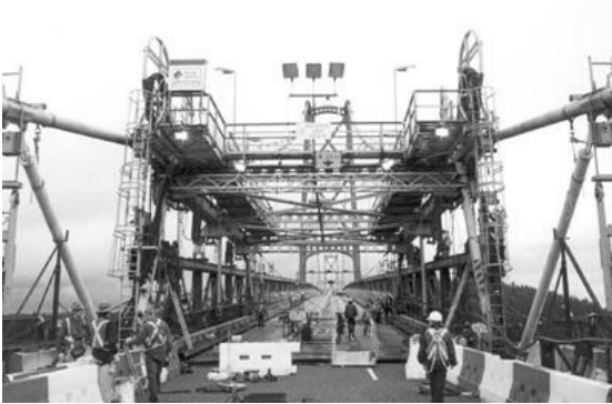
Lions Gate Bridge Deck Replacement
